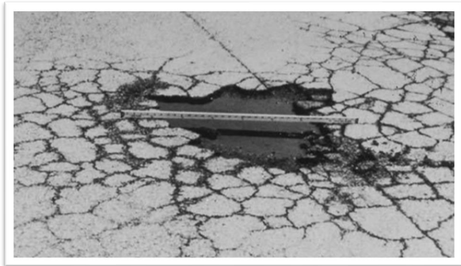
Figura N°44: Parches de Severidad Alta (H). Fuente: American Society for Testing and Materials, 2018
