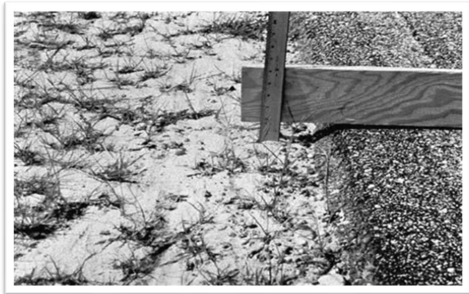
Figura N°32: Desnivel Carril – Berma con Severidad Baja (L) Fuente: American Society for Testing and Materials, 2018
