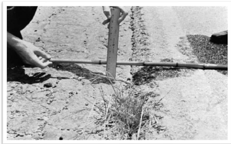
Figura N°33: Desnivel Carril – Berma con Severidad Media (M) Fuente: American Society for Testing and Materials, 2018
