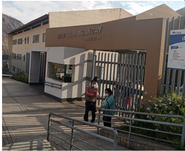
Hospital II de Abancay ESSALUD
