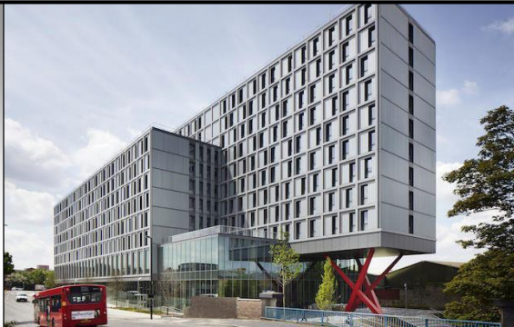
Figura N° 14 The Collective Old oak- Fachada Fuente: http://www.plparchitecture.com/the-collective-old-oak.html
