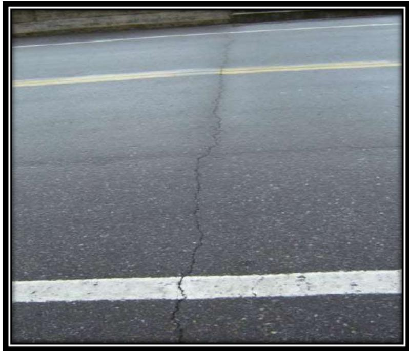
**Figura 12. Fisura Transversal**
