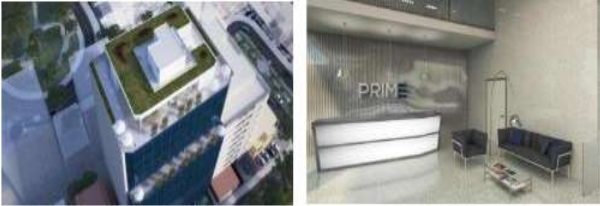
Figura 1: Edificio Prime Tower Magdalena
