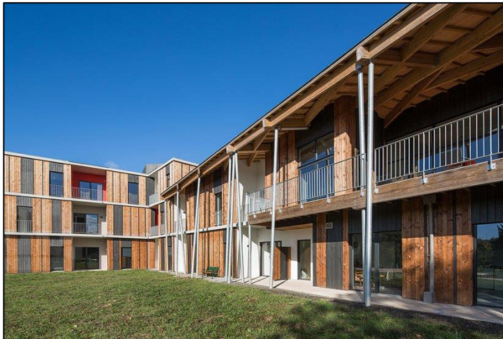
Figura 28: Exterior de la Residencia "Concoret Housing for the Elderly"
