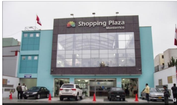
Figura 42. Fachada Shopping Plaza Monterrico
